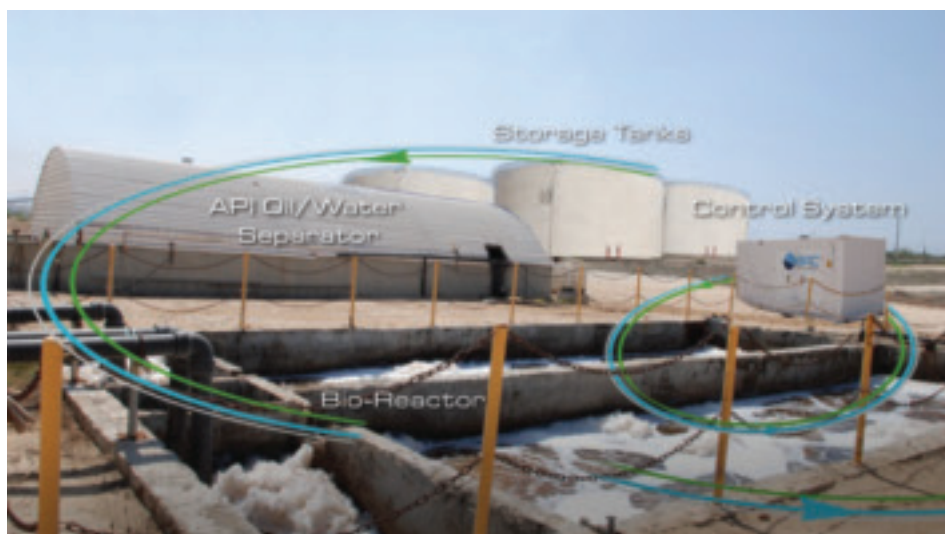
Figure 3: BPC integrates with existing infrastructure.
